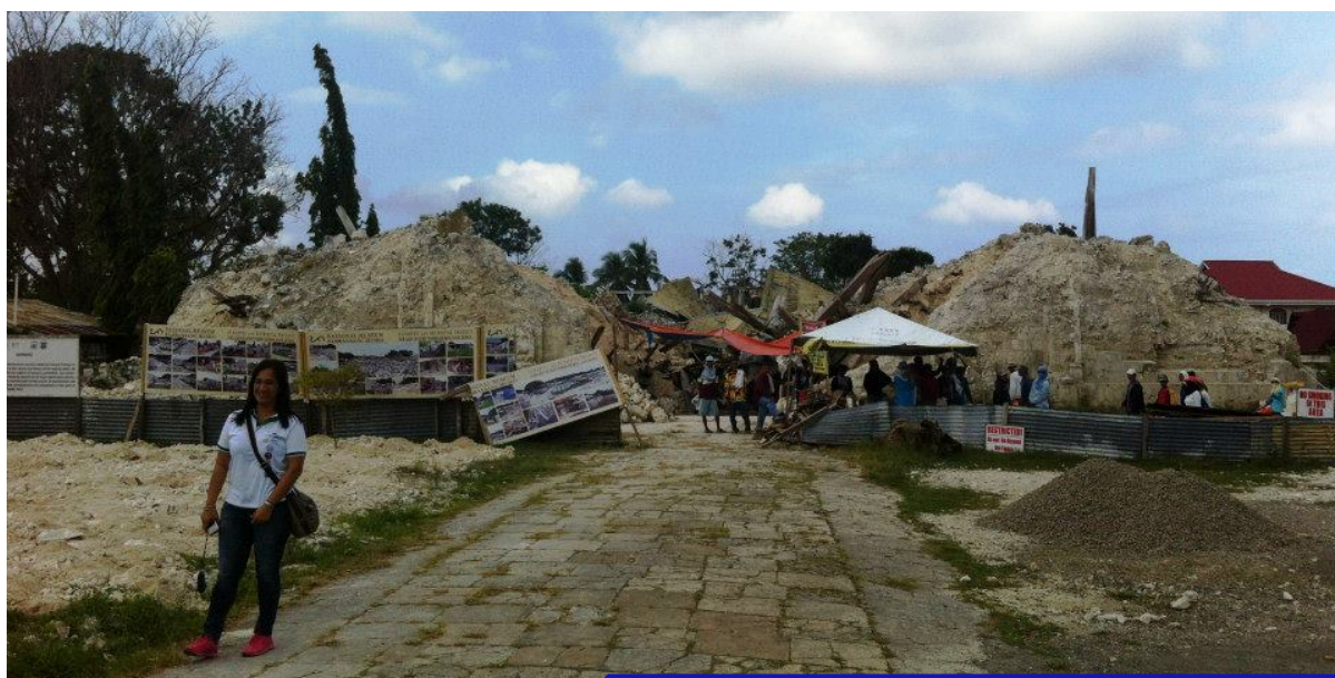
Ruins of Our Lady of Light Parish Church, a more than 100 year-old church in Loon, Bohol, which was destroyed by the 7.2 magnitude earthquake. Photo credits to Elmo Caralian
