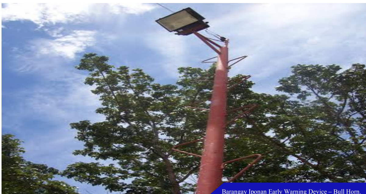
Barangay Iponan Early Warning Device – Bull Horn. Photo Credits to Cagayan De Oro LGU
